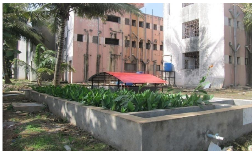
Wastewater treatment in the phytoremediation tank
