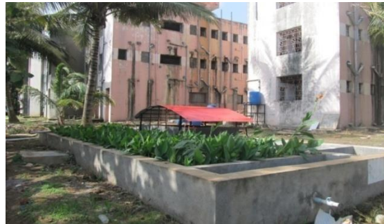
Gray water treatment plant at RIT
