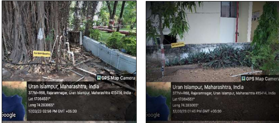
Fig 6: Rainwater harvesting units at College Campus
