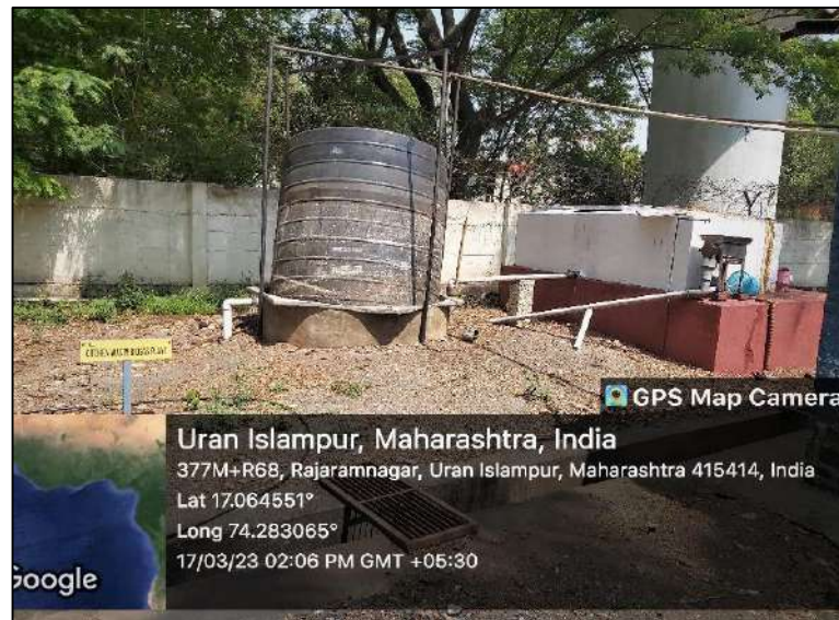
Fig 6: Biogas Plant near Boys Hostel
