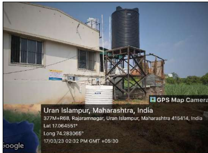
Fig 8: Laundry Waste Water Treatment Plant
